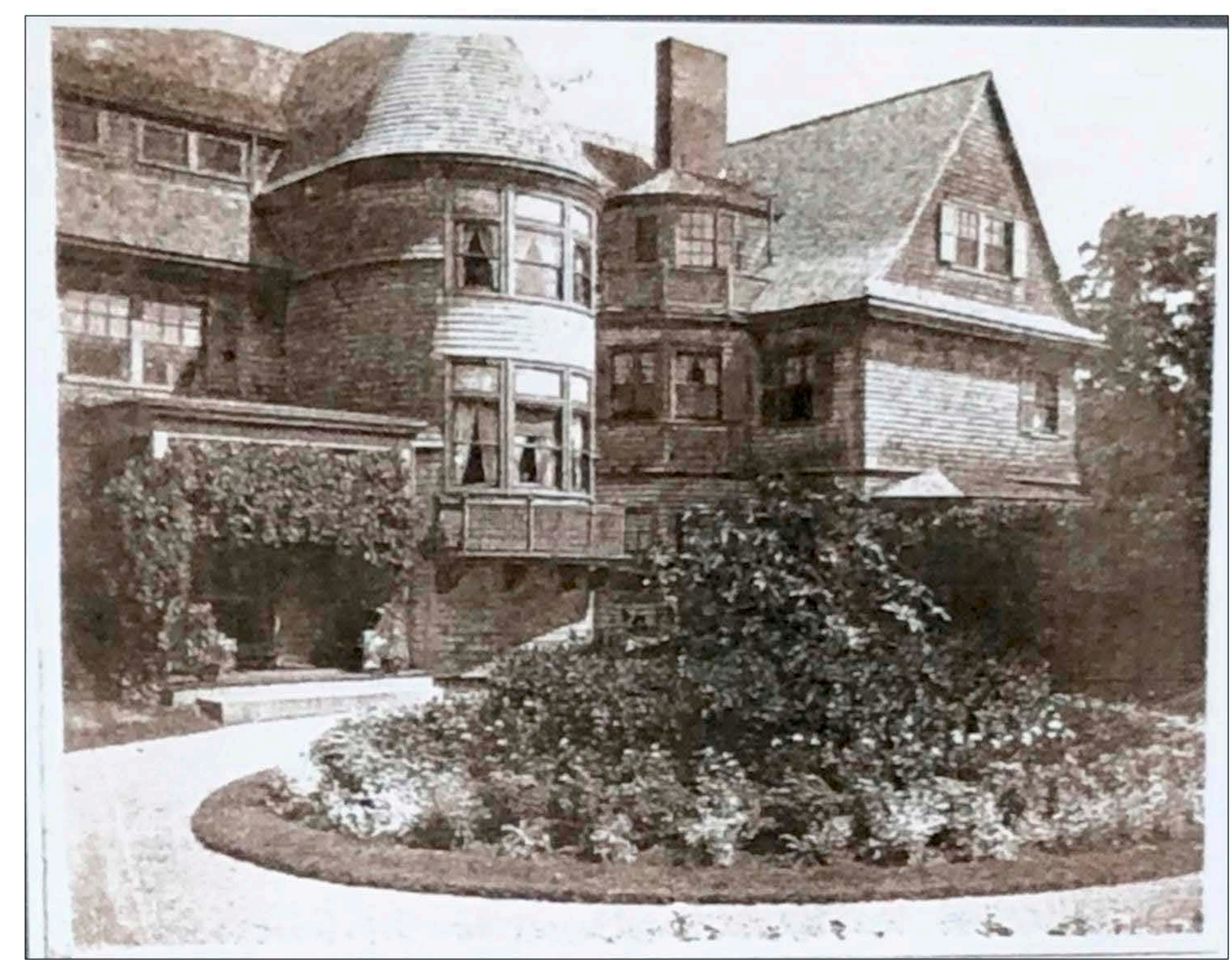
ORIGINAL HOUSE ENTRANCE
